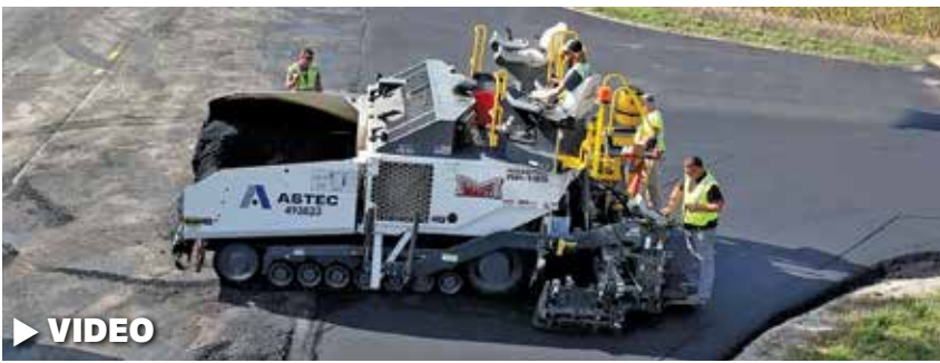
A Manatt's crew uses a Roadtec RP-195 paver from Astec to pave along Highway 30 near Jefferson, Iowa.
