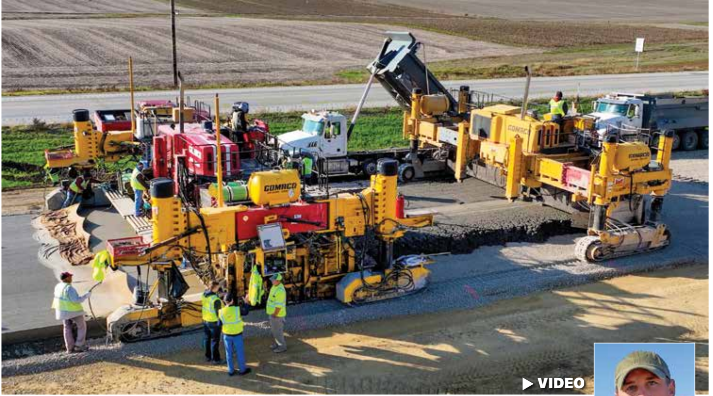
Manatt's uses a GOMACO GP-2600 slipform paver (left) and a GOMACO GHP-2800 slipform paver to build the westbound lane of Highway 30 near Atkins, Iowa. "We're pouring 30-foot wide by 10-inches thick, and we are aiming for 3,400 yards per day," said Roy Piper III, PCC Paving Superintendent. "To have the precision with the stringless technology simplifies everything."
