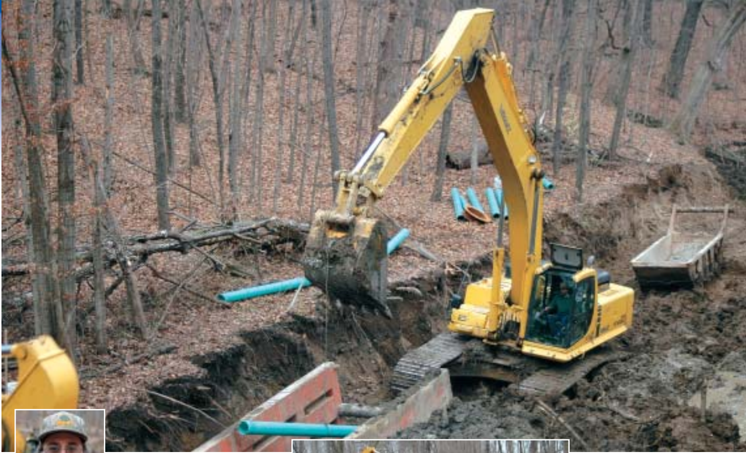
Operator Tim Brandt uses Valley Construction's Komatsu PC400LC-6 excavator to install 4,500 feet of sanitary sewer lines at the Rapids City housing development.
